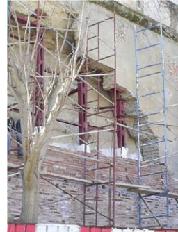
Fig.20- View of external wall during its restoration ©Abdessemed-Foufa 2006
