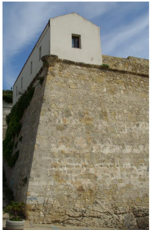
Fig. 4- North west sector of the bastion of Santa Croce
