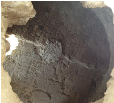
Fig. 8- Internal view of Porto Scudo Tower (Elena Cannas, 2014)
