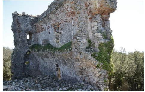
Fig. 6- Fortress of Giove - The interior façade, with the remains of the vaulted ceiling (A. Mancuso 2017)
