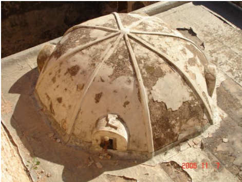
Fig. 2- Octagonal-based dome covering the bath (Serir, 2006)
