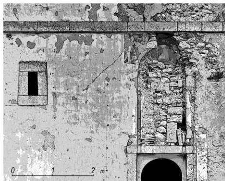
Fig. 9- Detail of the W side with the retractable bridge traces in the wall above the entrance.
