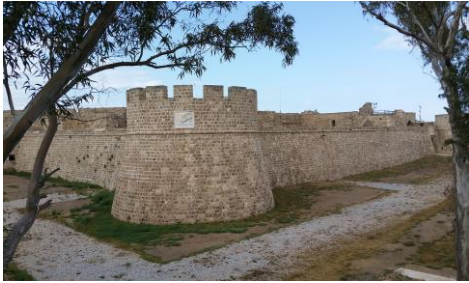
Figure 2 Othello's Tower after conservation work by UNDP PFF (Eppich, 2017)
