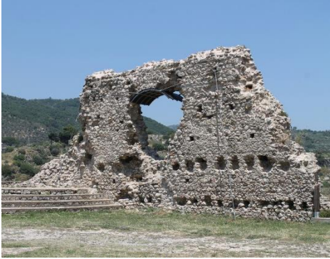
Fig. 9 Belcastro (CZ). The structure which supports the masonry above the heart-shaped gap.
