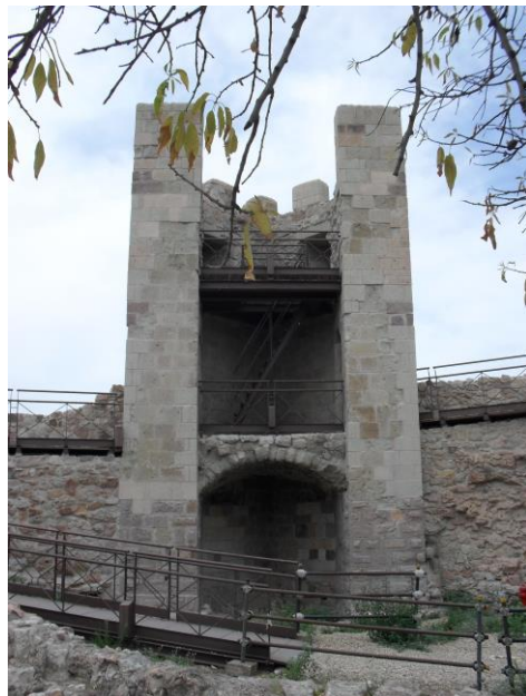
Fig. 3- East facade of pentagonal tower (view from inside of the castle)
