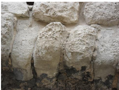
Fig. 4- Altered ashlar of inner vault of pentagonal tower (east facade) and the bedding mortars
