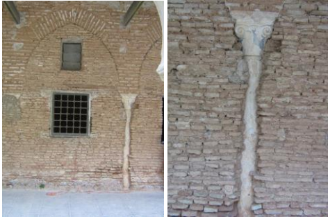
Fig.6a,6b- Column of the gallery enclosed in the bricks wall © Abdessemmed-Foufa 2006
