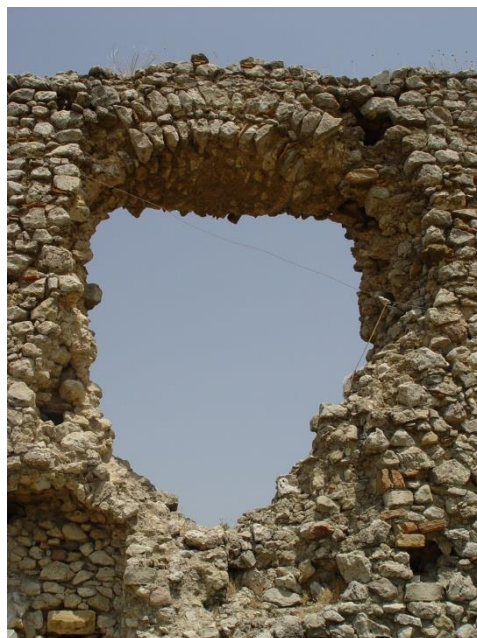
Fig. 4 Belcastro (CZ). The “heart” before the masonry reinforcement.
