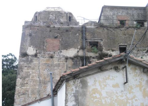
Fig. 2- the Music room built on rampart's platform (Archive of OGEBC)
